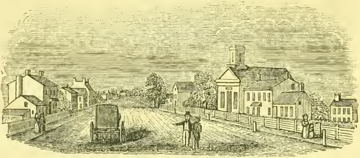
Central View in Middletown Point.
